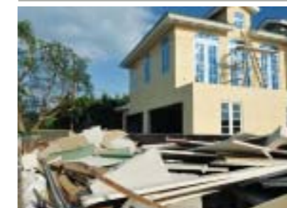
Onsite separation of wastes for recycling or reuse. (Source: Zero Waste WA)
