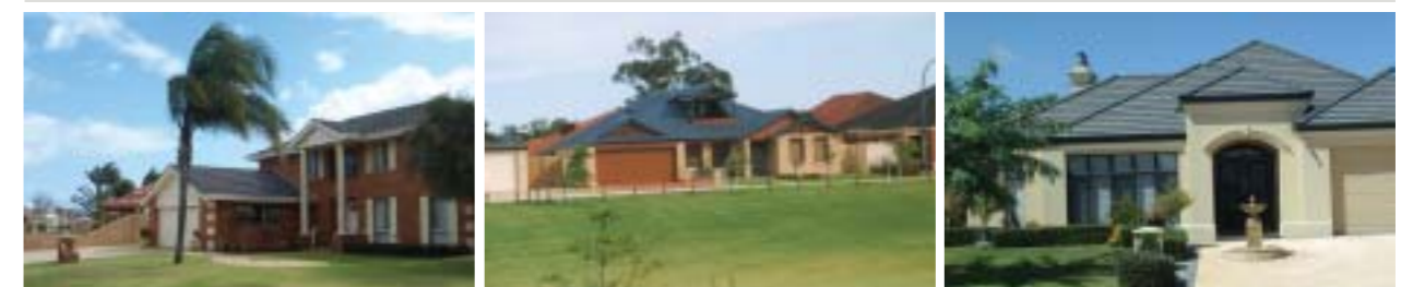
Dark roofs are exhibited. Colours are incompatible with 'Touch of White' colour palette.
